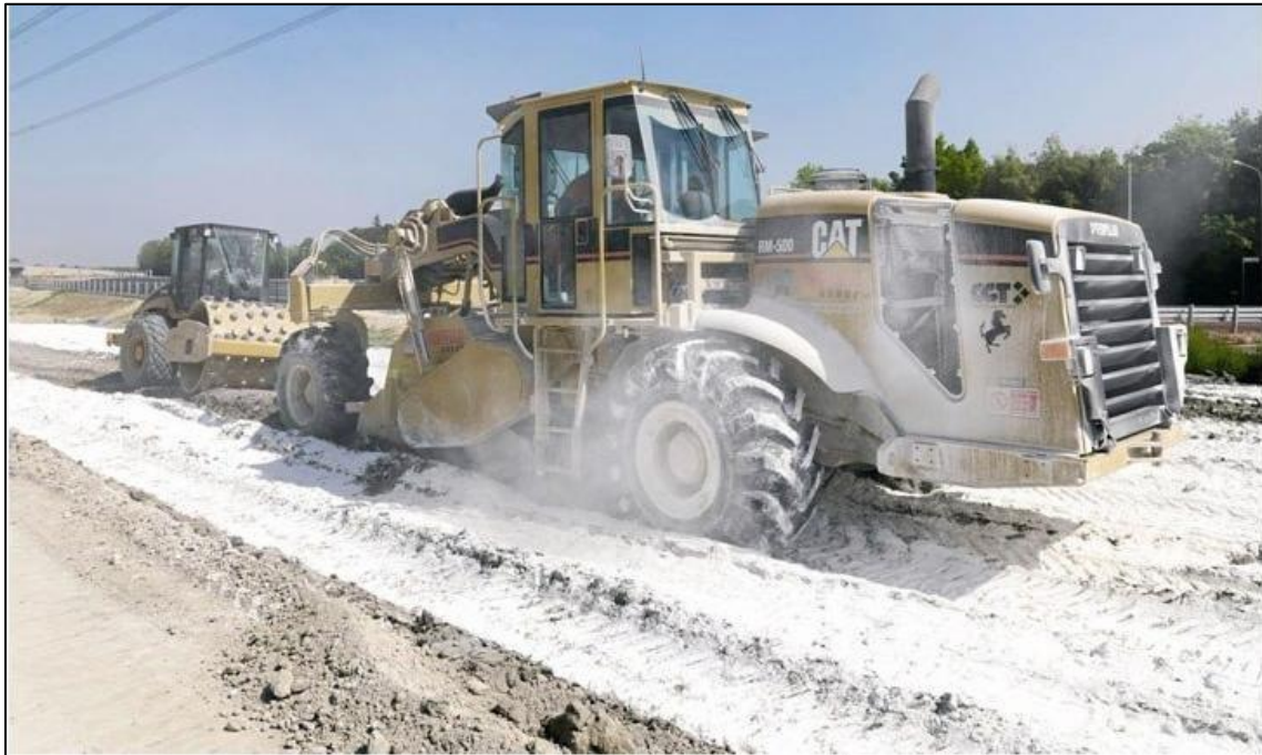
Figure 4. 5: Construction of a Lime stabilized low-volume rural road (Reference: Civilengineersforum )
