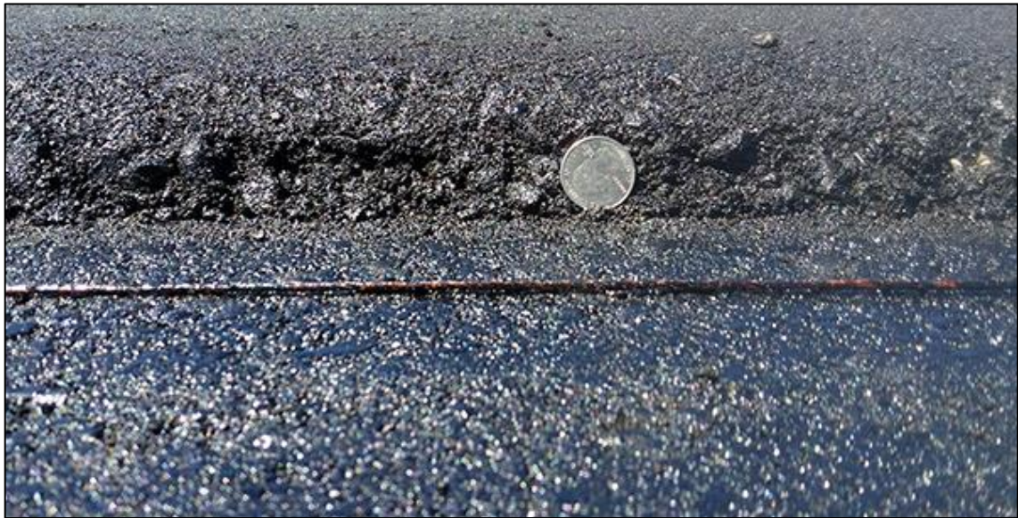
Figure 4. 14: Construction of a Thin bituminous surface (Reference : asphaltmagazine.com )
