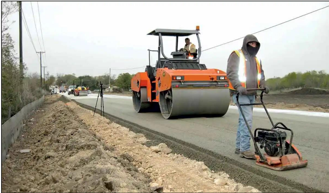
Figure 4. 15: Construction of a RCC low-volume rural road (Reference : Green Tech Programme )
