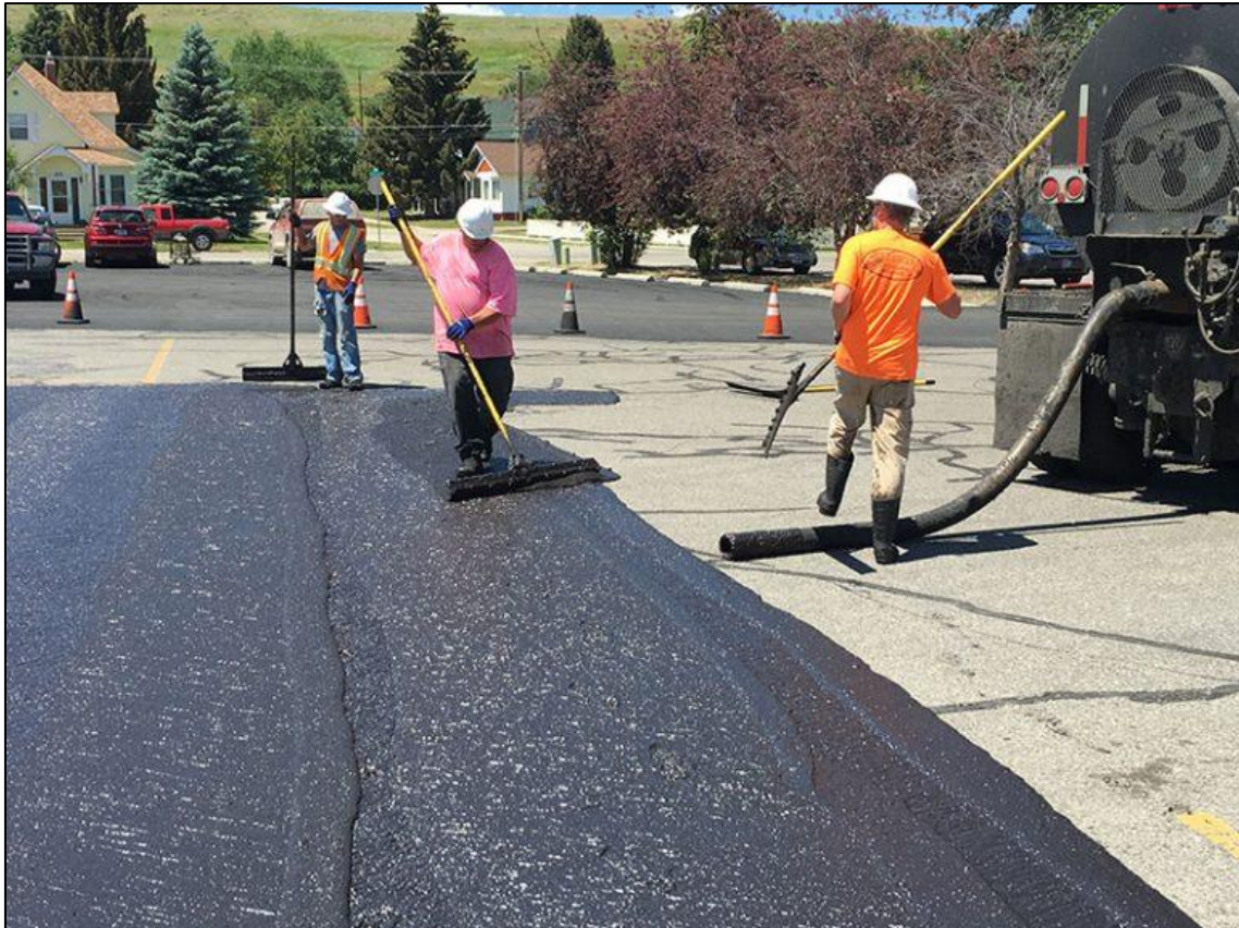
Figure 4. 9: Application of a Slurry seal low-volume rural road (Reference: Bitumen6070 )
