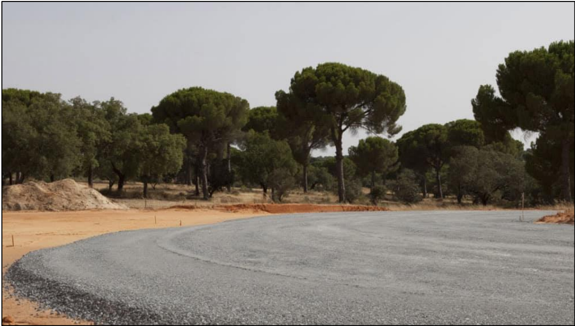
Figure 4. 6: Construction of a Bitumen stabilized low-volume rural road (Reference: Globalroadtechnology )
