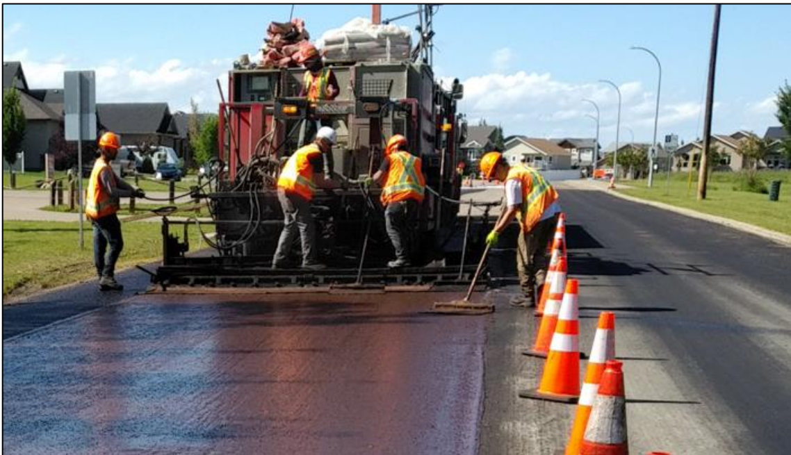
Figure 4. 8: Application of a Microsurfacing low-volume rural road (Reference: Red Deer )
