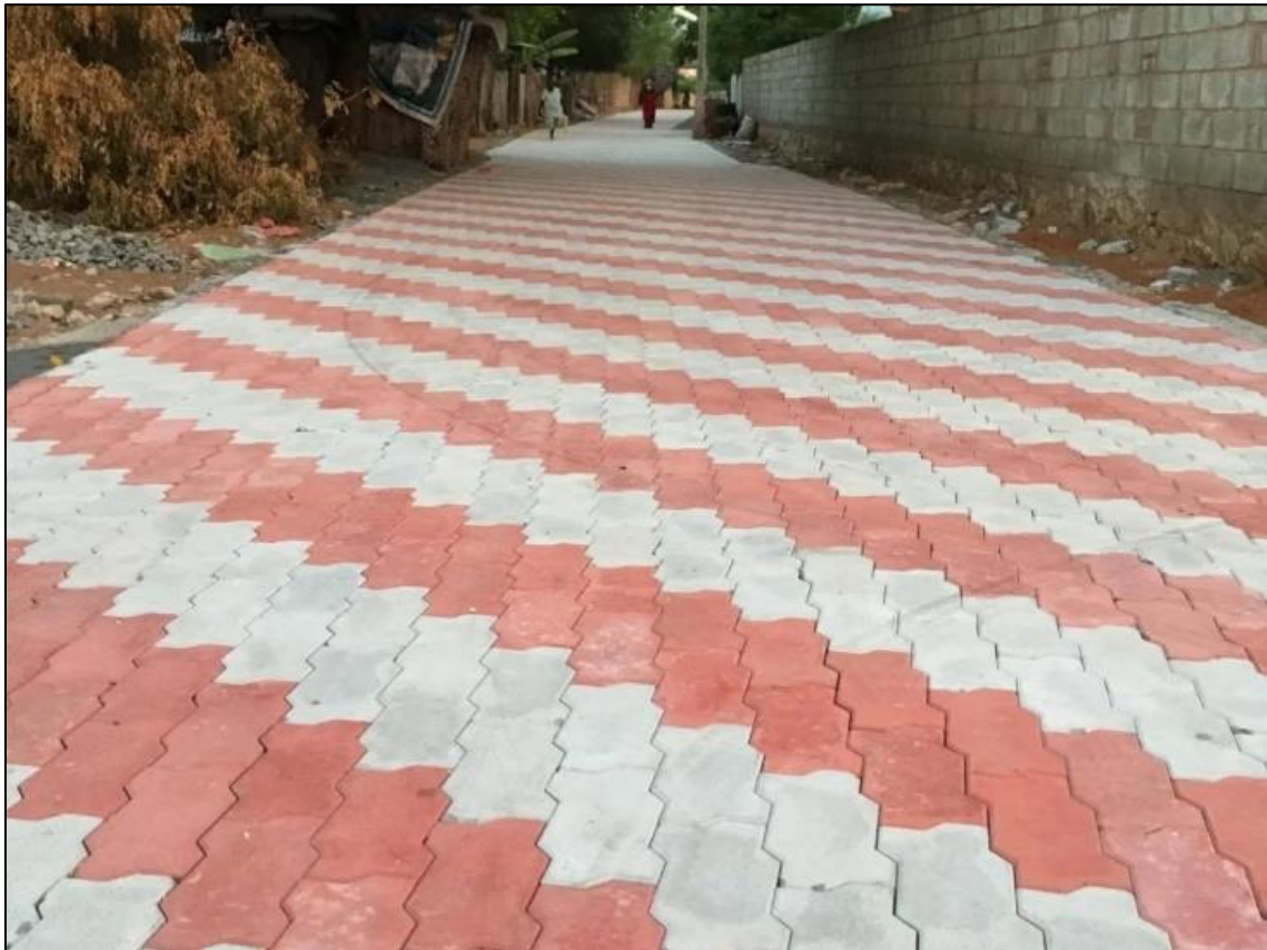
Figure 4. 13: Concrete paving block pavement (Reference : Jontypavertiles )
