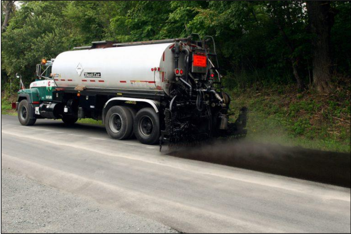
Figure 4. 10: Application of a Fog seal low-volume rural road (Reference : Rahabitumen )
