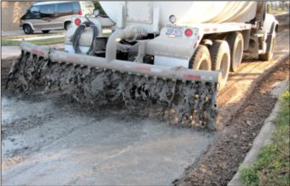
Figure 4. 4: Construction of a Cement stabilized low-volume rural road (Reference: Matinmarietta )
