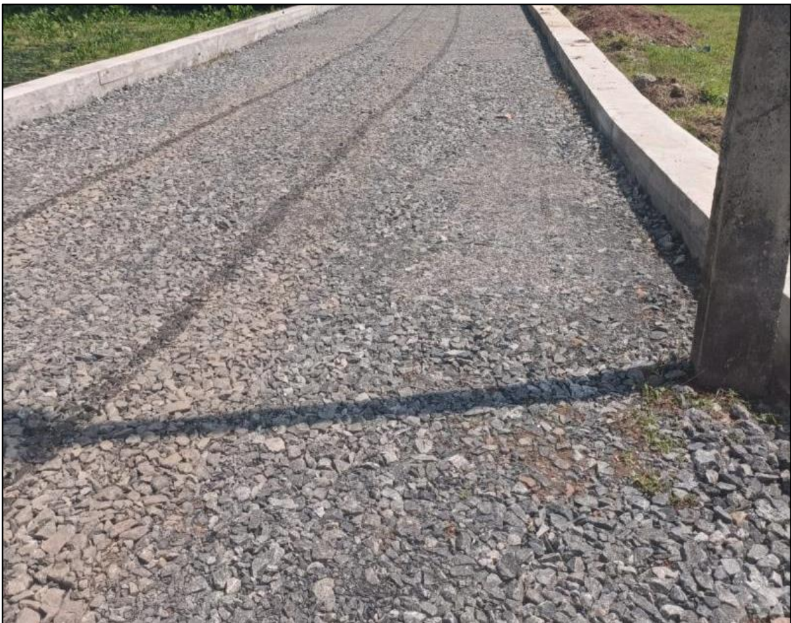
Figure 4. 3: Wet Mix Macadam Road (Reference: Rebuild Kerala Initiative )
